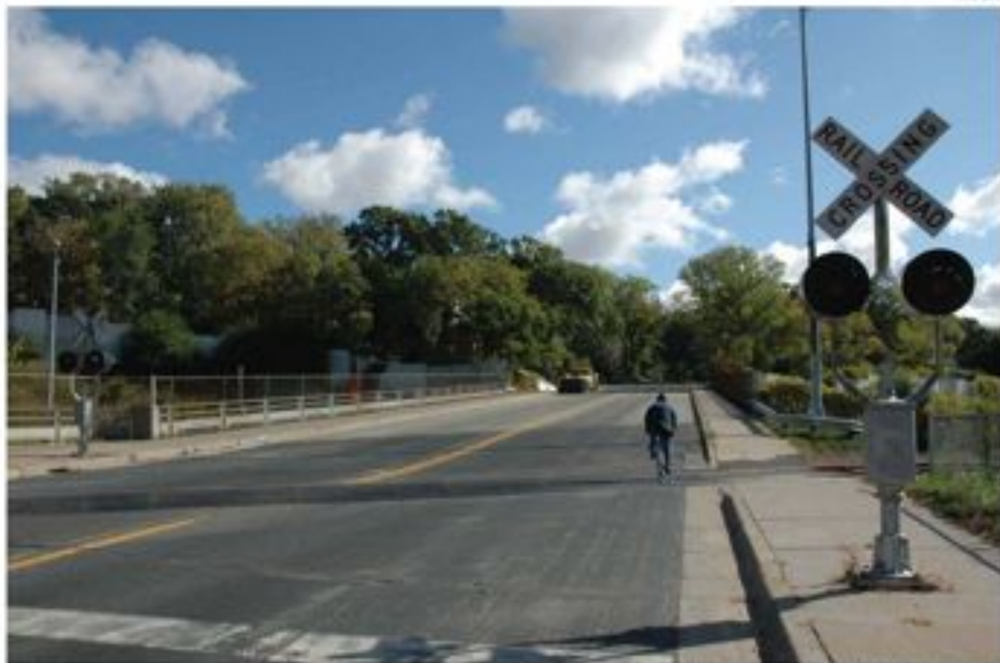
Franklin Avenue Bridge over Interstate 94 looking east Image compliments of The Metropolitan Design Center
