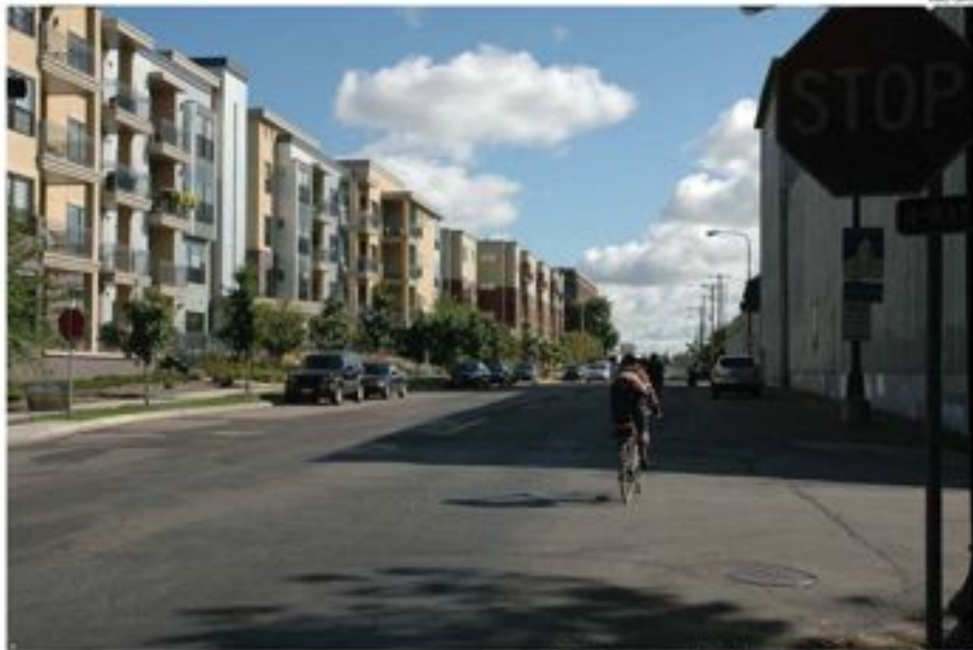
Franklin Avenue looking east near Emerald Street Image compliments of the Metropolitan Design Center
