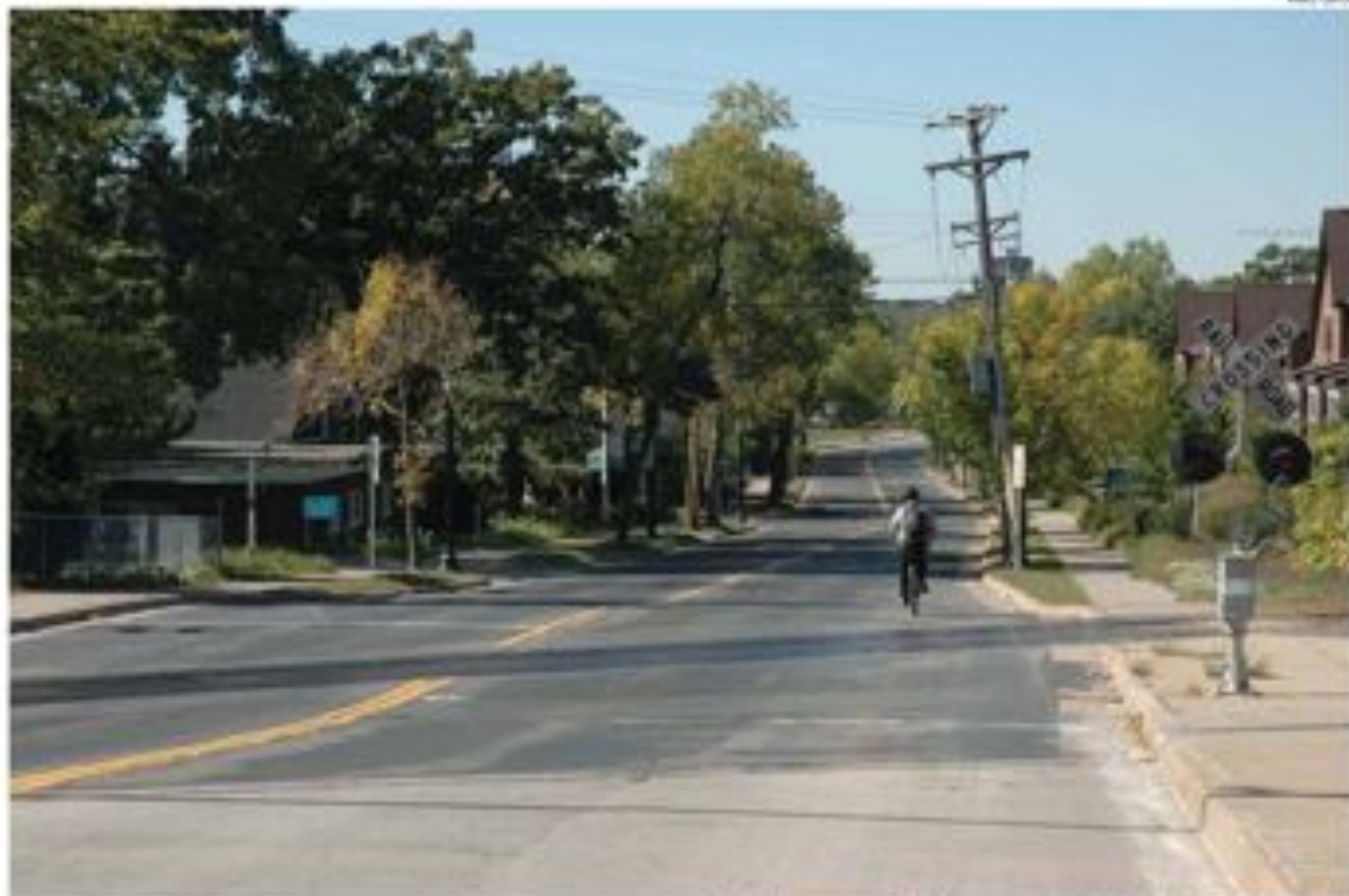
Franklin Avenue Bridge over Interstate 94 looking west Image compliments of the Metropolitan Design Center
